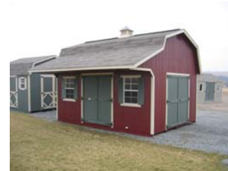
Barn with Porch
